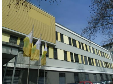
Post retrofit Source: IWU
