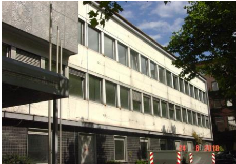
Before retrofit Source: IWU
