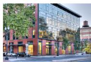
renovation and 50% new construction, with a seismic retrofit acting as the "knuckle" between existing and new. The four-story building (with one floor below grade on the existing portion) includes corporate offices on the upper floors and a global learning center on the ground floor. Mercy Corps describes its new headquarters were the production of the
