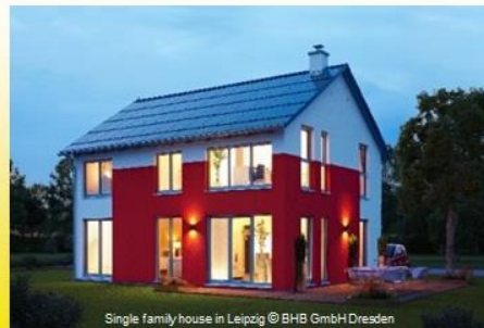
Single family house in Leipzig © BHB GmbH Dresden
